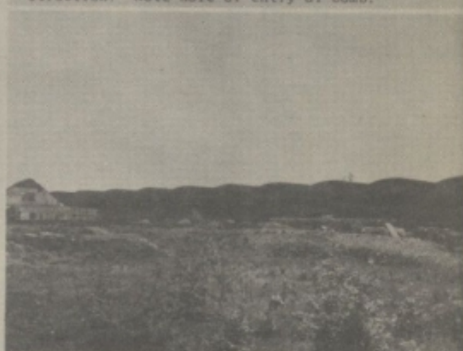
Photo 7 - Allach - Completely destroyed canteen in foreground. Several bays of large assembly hall in background.
