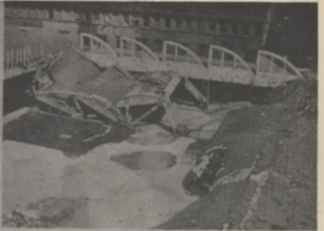
Photo 12 - Oberwiesenfeld - General view of area where collapse due to blast occurred.
