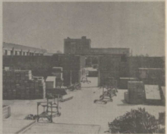
Photo 20 - Allach - Bldg destroyed by fire. Walls left standing.
