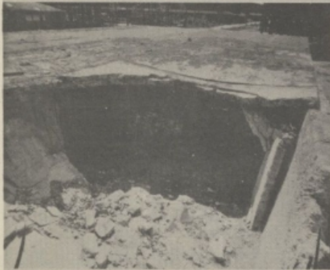
Photo 19 - Allach - Same as 14, showing top of bldg 2091.
