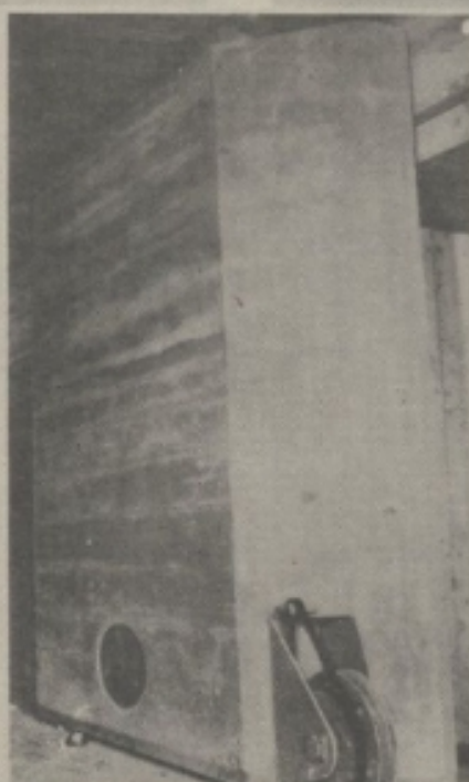
Photo 9 - Allach - Heavy door to bunker, closed during air attacks.
