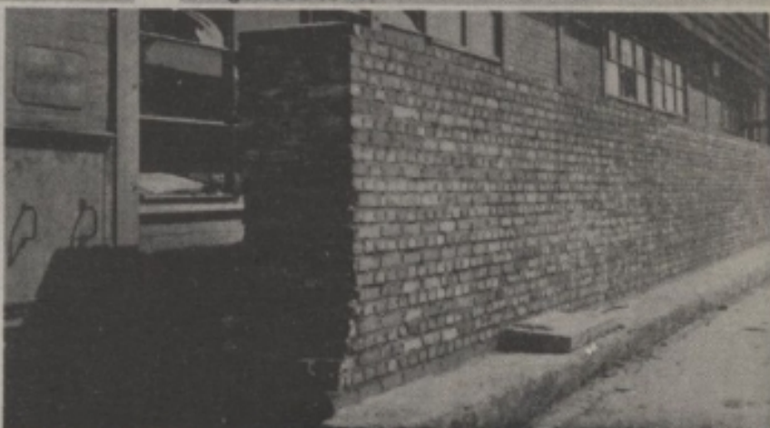
Photo 26 - Oberwiesenfeld. Heavy precast concrete blocks used to protect generator.
