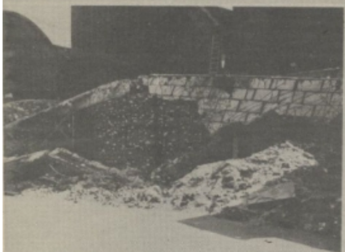
Photo 6 - Allach - New construction, 1940; new brick wall to isolate damaged portion.
