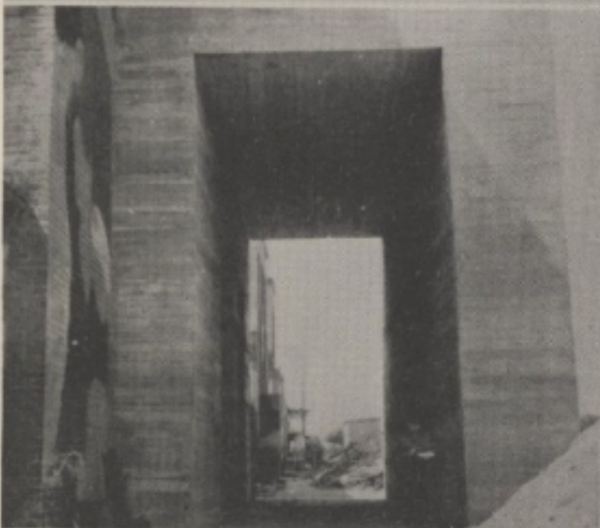
Photo 25 - Oberwiesenfeld. Heavy reinforced concrete structure to house transformer station.
