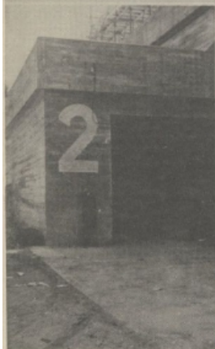
Photo 8 - Allach - Protection to entrance of bunker structure.
