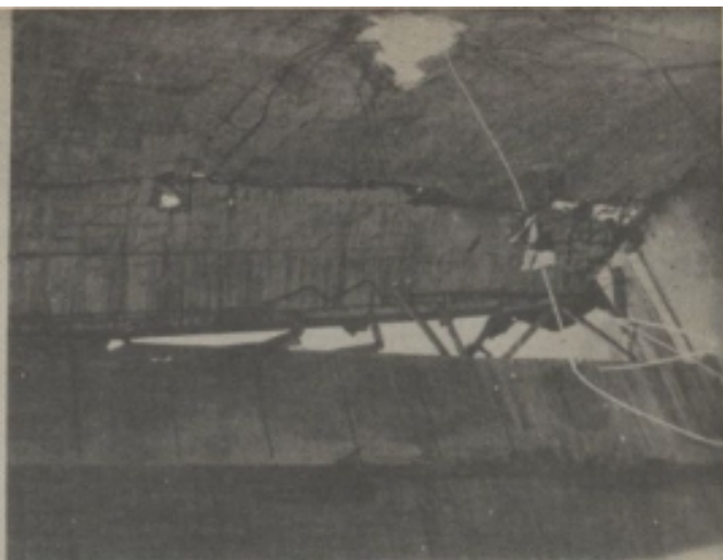
Photo 5 - Allach - New reinforced concrete construction. Note hole of entry of bomb.
