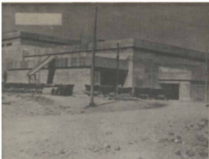
Photo 4 - Allach - Heavy bunker type construction used as a machine shop.
