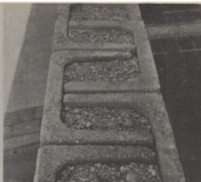
Photo 24 - Oberwiesenfeld. Top view of precast concrete blocks and gravel, used as blast walls.
