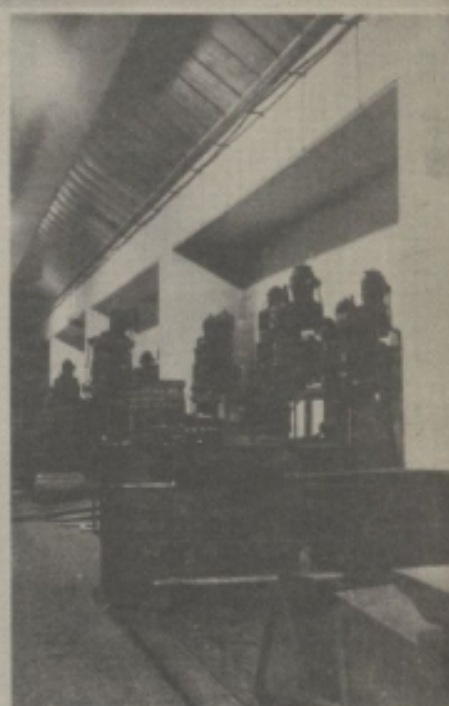
Photo 10 - Allach - Inside of bunker showing machine tools.
